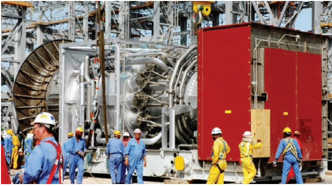
Turbine installation in 2006
