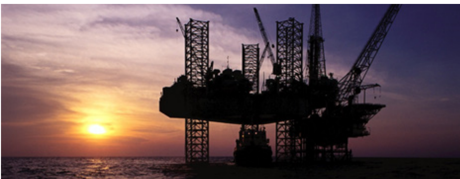
The One-Stage Sandstone Acid system remediated a struggling disposal well.
