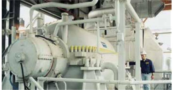
**Barrel** - Vertically-split barrel compressors are used primarily for high-pressure applications such as ammonia, urea and methanol synthesis, refinery recycle, natural gas compression and injection, and hazardous gases.
