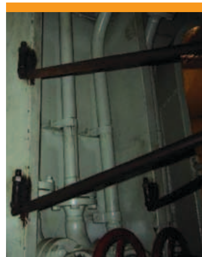
b) An example of transducer holder inside of a hydro-generator chamber: holder fixing to the chamber wall (top), and holder head – allowing non-contact transducer connection (bottom).
