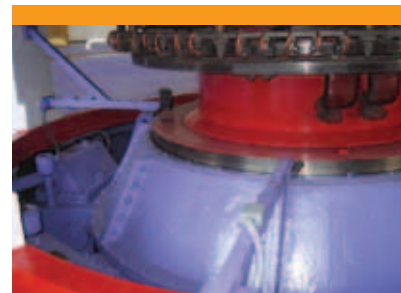
a) Two rigid bars holding non-contact transducers are connected to a static structure
