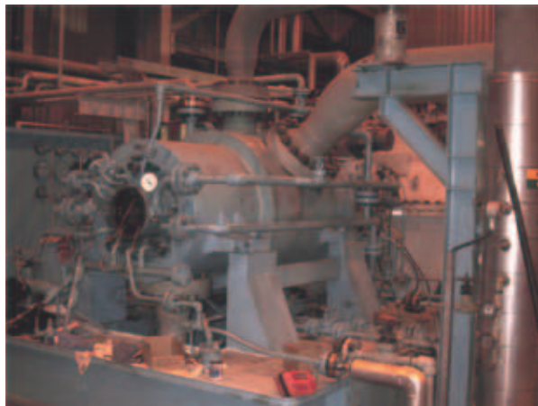
Synthesis Gas Compressor, High Pressure Case.
